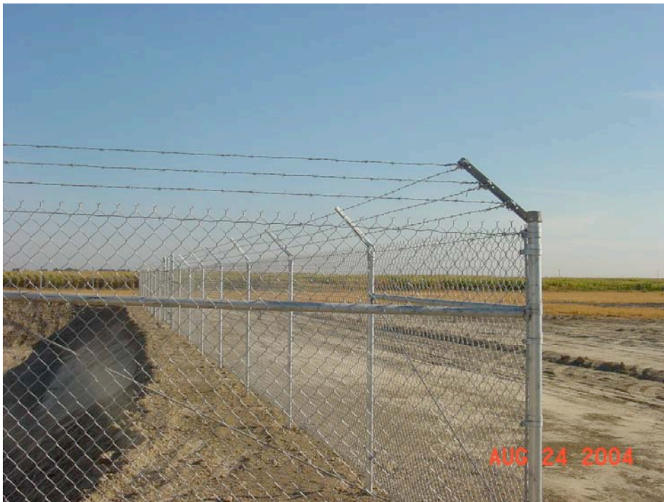
Picture 5. Fencing on the perimeter of the dairy like this chain-link fence will prevent the entry of people or animals into the livestock housing areas. Appropriate separation is still required to prevent items from being thrown into cow corrals.
