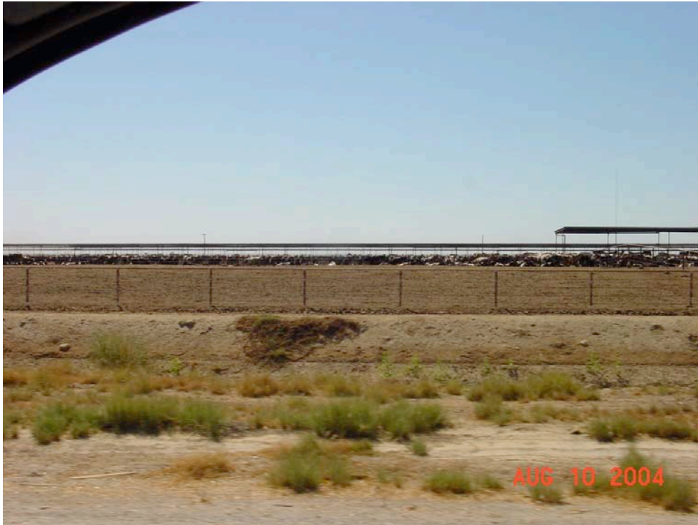
Picture 1. Typical pipe fence with cable wires. Note that in the top picture there is an irrigation ditch between the roadway and the fencing that will provide some protection from direct access to corrals.
