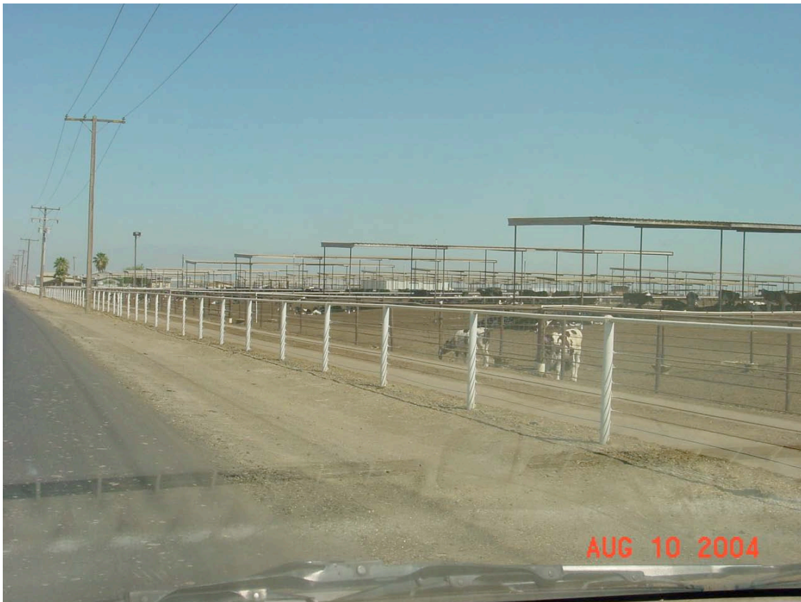
Picture 3. Perimeter fencing with a space barrier between the perimeter fence and livestock corral fence. In this particular case, the space barrier is too small to prevent anyone from throwing objects into the calf corrals.
